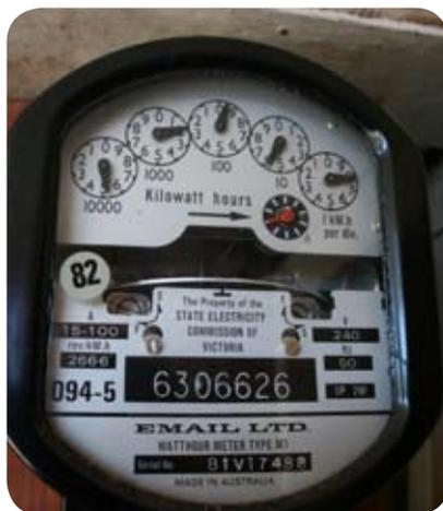
To read a meter with a clockface, begin by standing directly in front of the meter. Commence reading from the right hand side, reading the dials in turn – ABCDE. Write down the corresponding figures from right to left as read.
